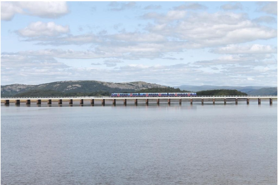
Arnside Viaduct – 14 th July 2015
